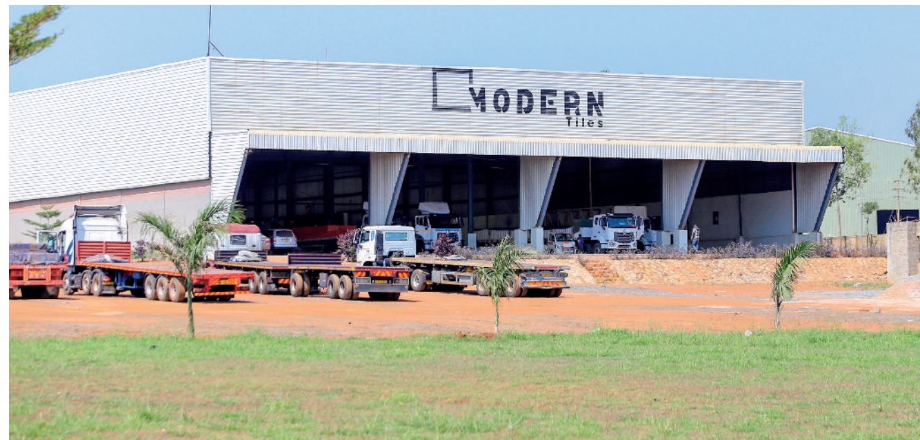
Modern Tiles Limited factory
